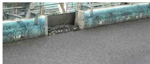
The plant had historical foaming problems. A 20 cm foam board was a permanent feature.
