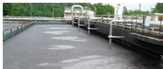
Picture taken two weeks after commencing sludge ozonation. The foam is gone and the liquid level in the basin is visible.
